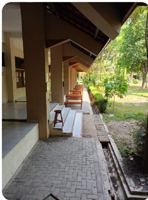
Paving keliling Kampus III Paingan antara kantin-poliklinik
